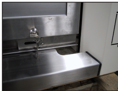
Sash lock down with key ensures that sash is not raised by unauthorized personnel.
